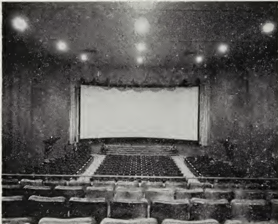
The screen in this 1400-seat house is 25 by 62 feet and was furnished by Raytone. Notice that the screen runs from wall to wall, with the complete elimination of traditional proscenium. Heywood Wakefield chairs are used.
